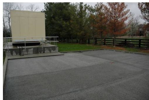
Pervious Concrete – After Rain Event – LFUCG South Elkhorn Pump Station
