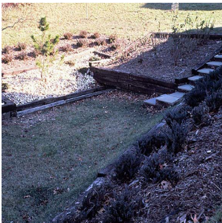
An Example of an Infiltration Basin
