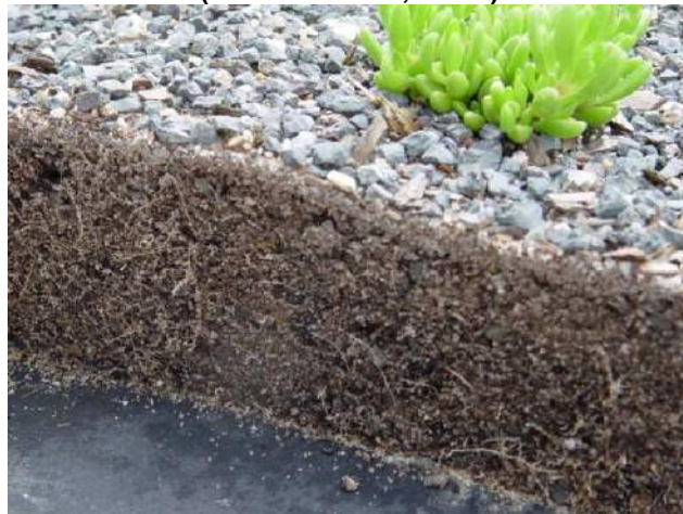
Figure 3 Photos of Vegetated Roof Cross-Sections (source: B. Hunt, NCSU)
