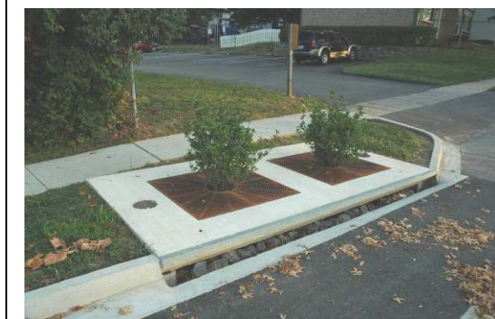
Tree Box Filter – Gainesway Pond, Lexington, KY
