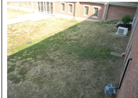
Downspout disconnection
