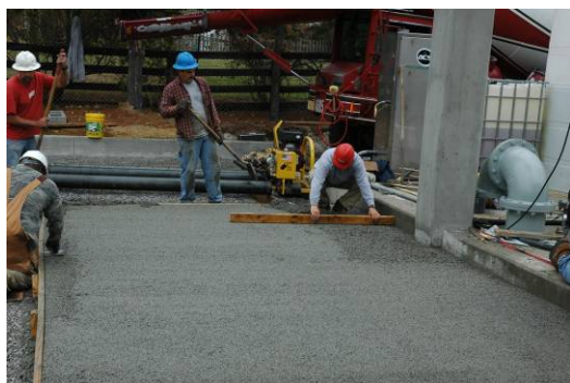
Pervious Concrete – During Placement
