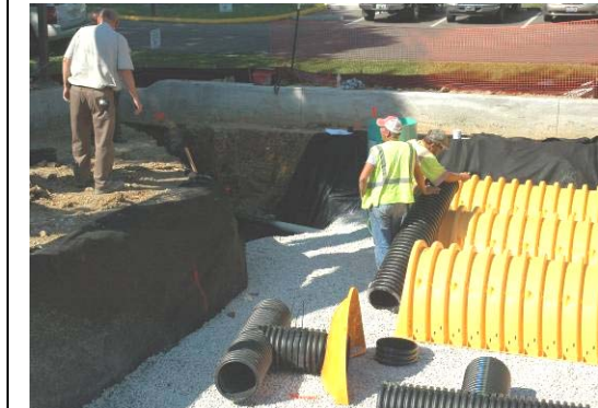
Underground Stormwater Storage-detail
