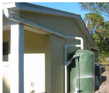
Rain Barrel - Commercial
