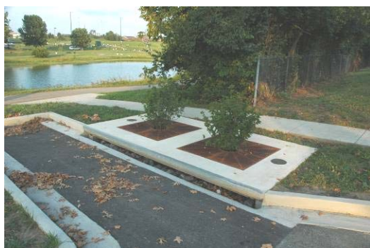
Tree Box Filter – Gainesway Pond, Lexington, KY
