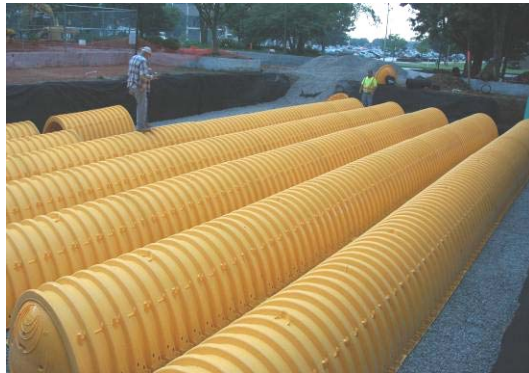
Underground Stormwater Storage
