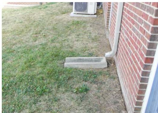
Downspout disconnection
