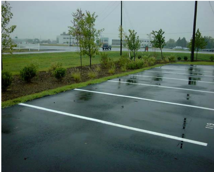
Bioretention Basins in office setting parking lot.
