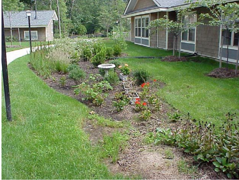
Bioretention Filter in multi-family residential setting.
